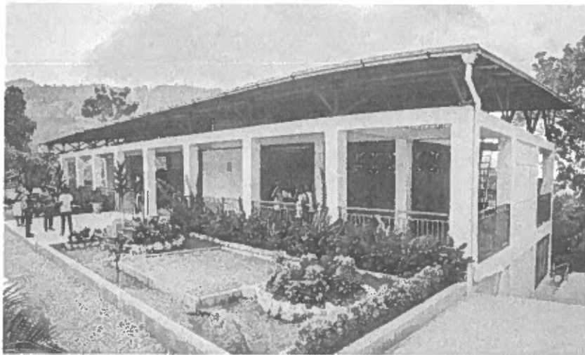
Fig. 5. Haiti Partners' school building, with its earthquake resistant, open-air design, houses two large classrooms upstairs, and a health clinic, pharmacy, and offices on the lower level.
